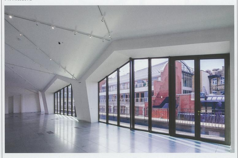
Above The new folded mansard roof, styled on Bacon's studio, has created a ceiling of sloped planes
